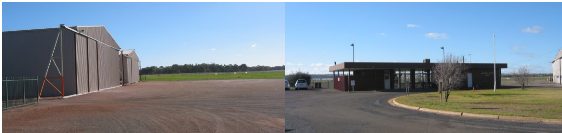
Figure 8-6: Narrandera airport and hangar facility.
